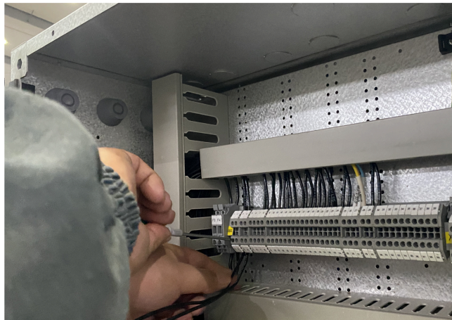
figure 7-3 XSG terminal block
