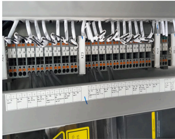
figure 7-2 SCU terminal block
